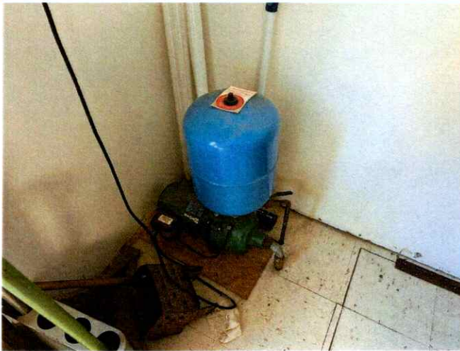
Well water pump assembly
