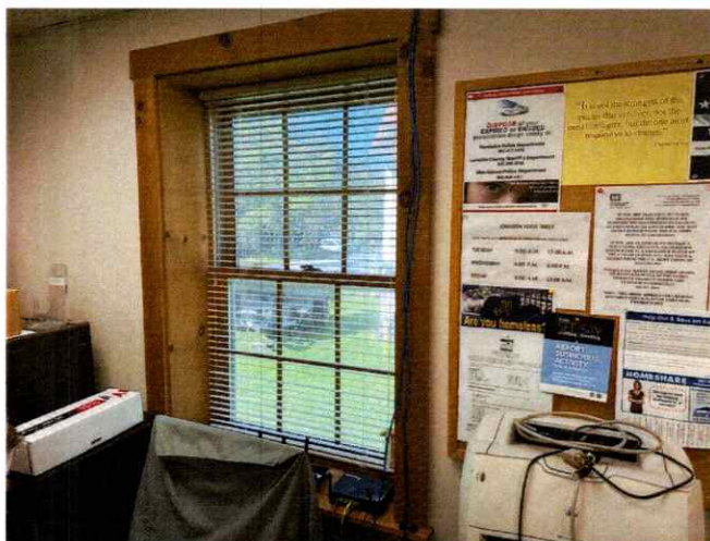
Typical double hung window, wood frame, double pane
