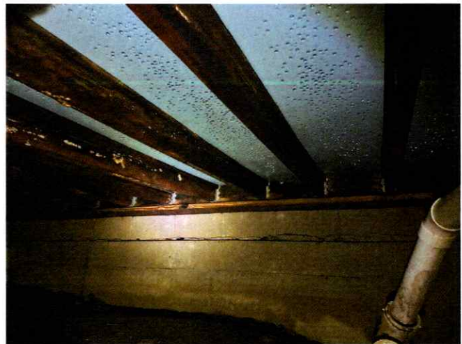
Underneath building addition, showing two (2) inch blue foam insulation between rafters. No tag or R value visible
