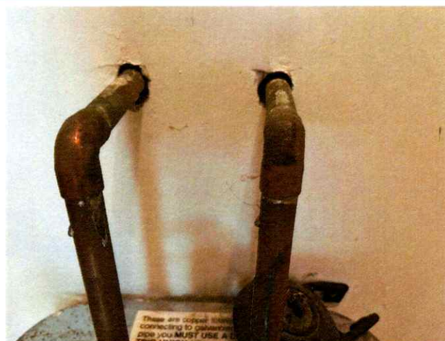
Copper plumbing penetration from the well pump and tank, to the water heater
